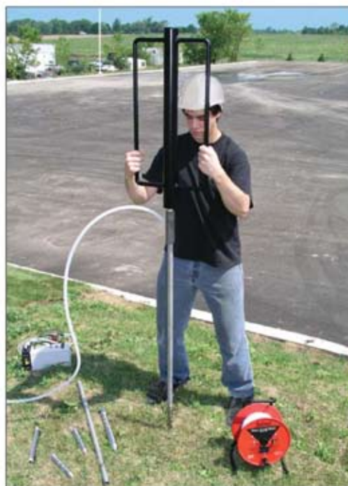
Installing Piezometers with a Manual Slide Hammer
